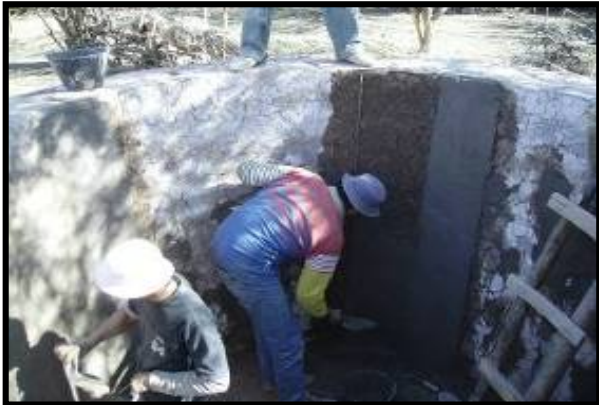
Vista del revoque impermeable al interior
