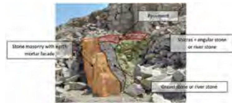
Fig.3 The first type of nucleus structure in La Galería pyramid (credits: J. Vargas-Neumann)
