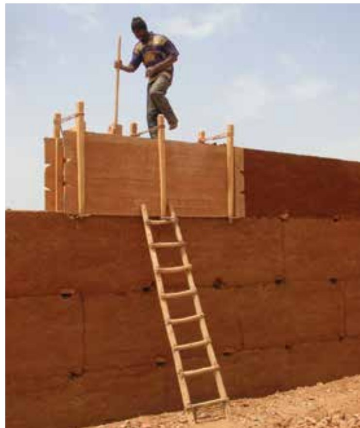
Fig.4 Rammed-earth masonry construction in the Drâa Valley (credits: Saverio Mecca, 2007)
