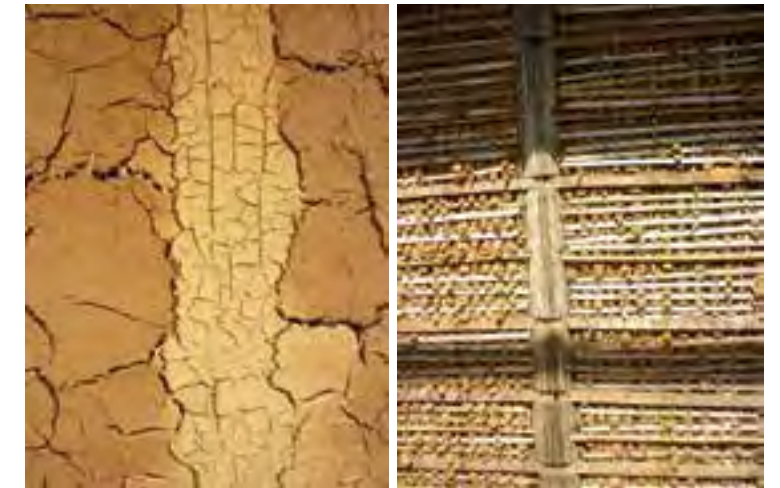
a) Shrinkage fissures resulting from drying of the first earthen layer; Fig.4a) b) Appearance of the inboard side (credits: Akemi Hijioka, 2010)
