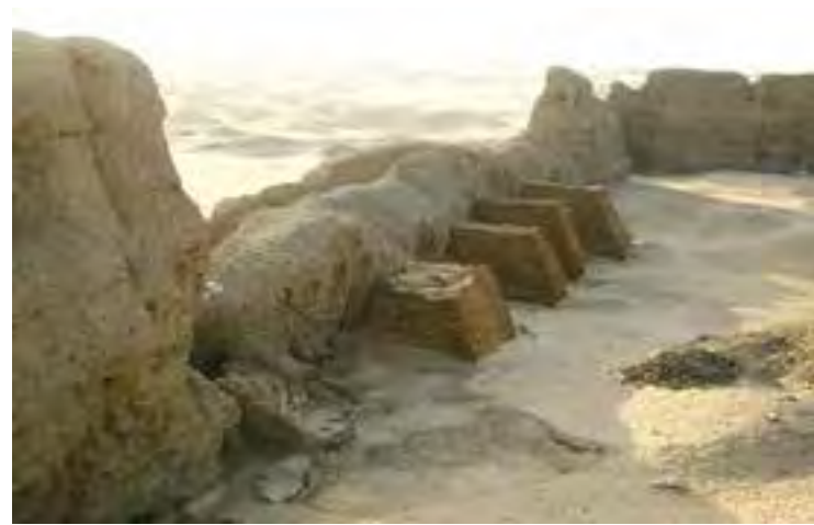
Fig.2 Large sandbag buttresses were constructed in 2001 to support the east enclosure wall (credits: Anthony Crosby, 2006)
