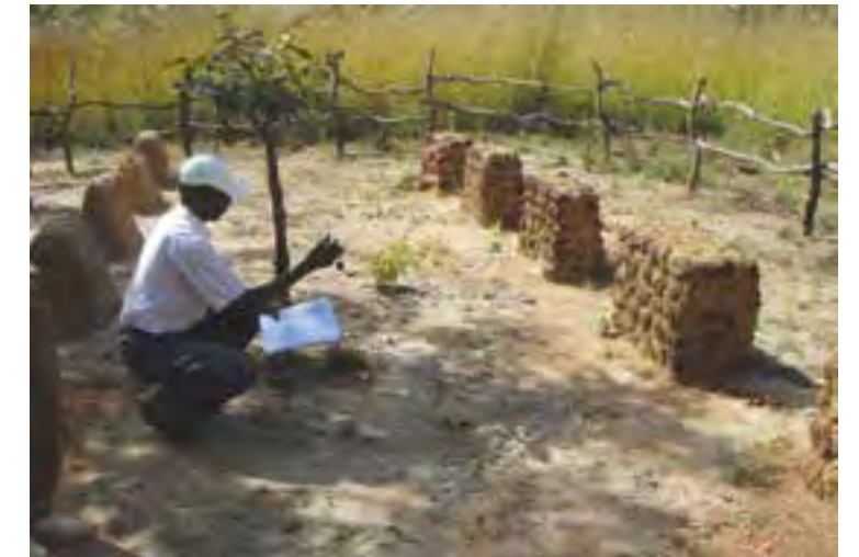
Fig.6 Preventive measure with sacrificial capping, Fayaz Tepa, UNESCO-Japan-Fund-in-Trust project, Uzbekistan (credits: Thierry Joffroy, 2003)
