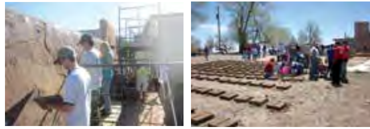
Fig.3 Volunteers plastering walls at San Miguel Chapel in Santa Fe, NM (credits: Jake Barrow, 2011)
