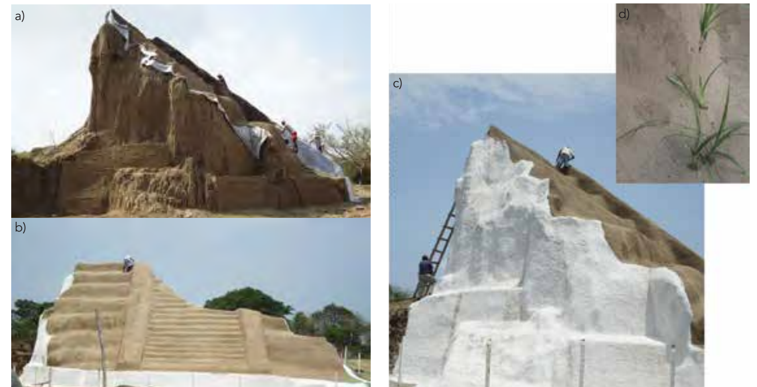
Fig.5 La Joya Pyramid in spring 2009: first preservation experiment: a) retaining walls at the foot of west façade and on the north profile, placing of geotextile and protective layer; b) west façade after preservation; c) north profile after preservation and d) weeds growing through geotextile and sacrificial layer (credits: Annick Daneels, from project authorized by the Archaeology Council of Mexico's National Institute of Anthropology and History)
