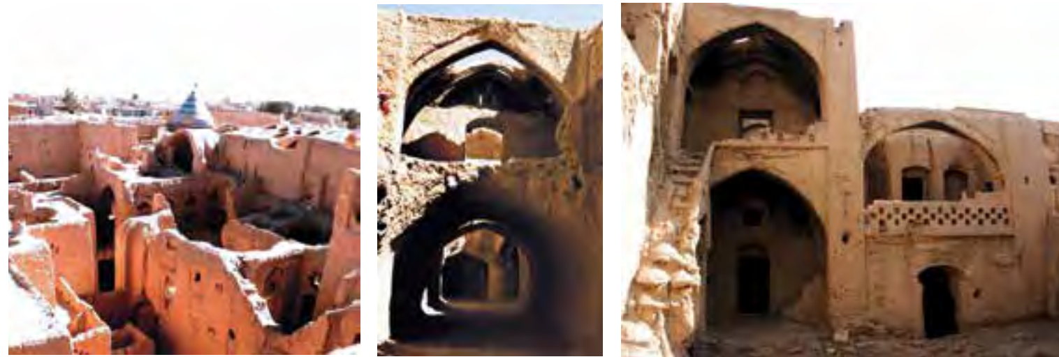
Fig.2, Fig.3 and Fig.4 Historical structures in Moorcheh Khort, Iran (credits: M. R. Manouchehri, 2008)
