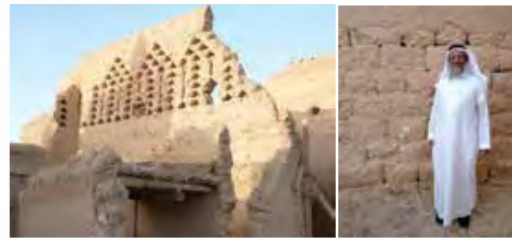
Fig.2 A wide variety of historic Najdi architecture is found on the site (credits: Pamela Jerome, 2011)
