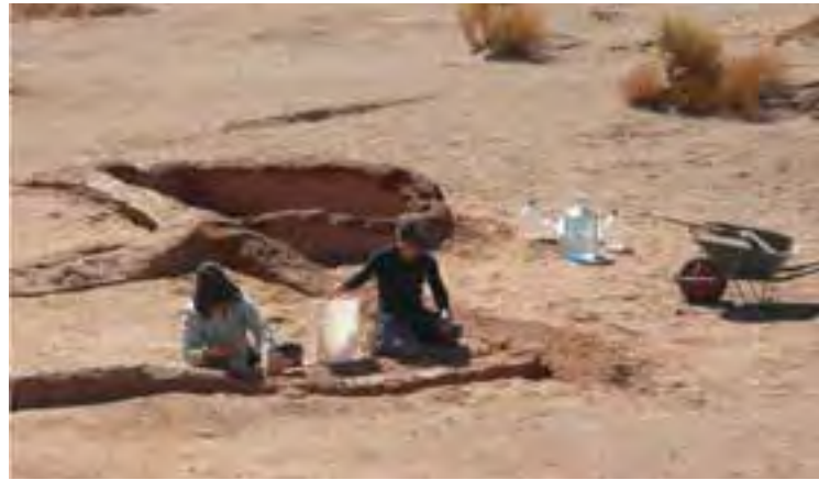
Fig.3 Removal of salt-contaminated first coating layer. (credits: Monica Bahamondez)
