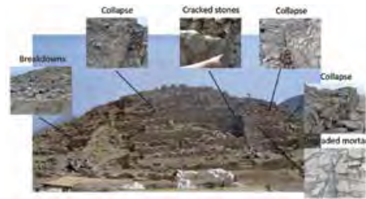
Fig.1 La Galería Stepped Pyramid, Caral, Peru, constructed of stone and earth around 2700 BCE. Signs of deterioration (credits: J. Vargas, C. Iwaki, A. Rubiños)
