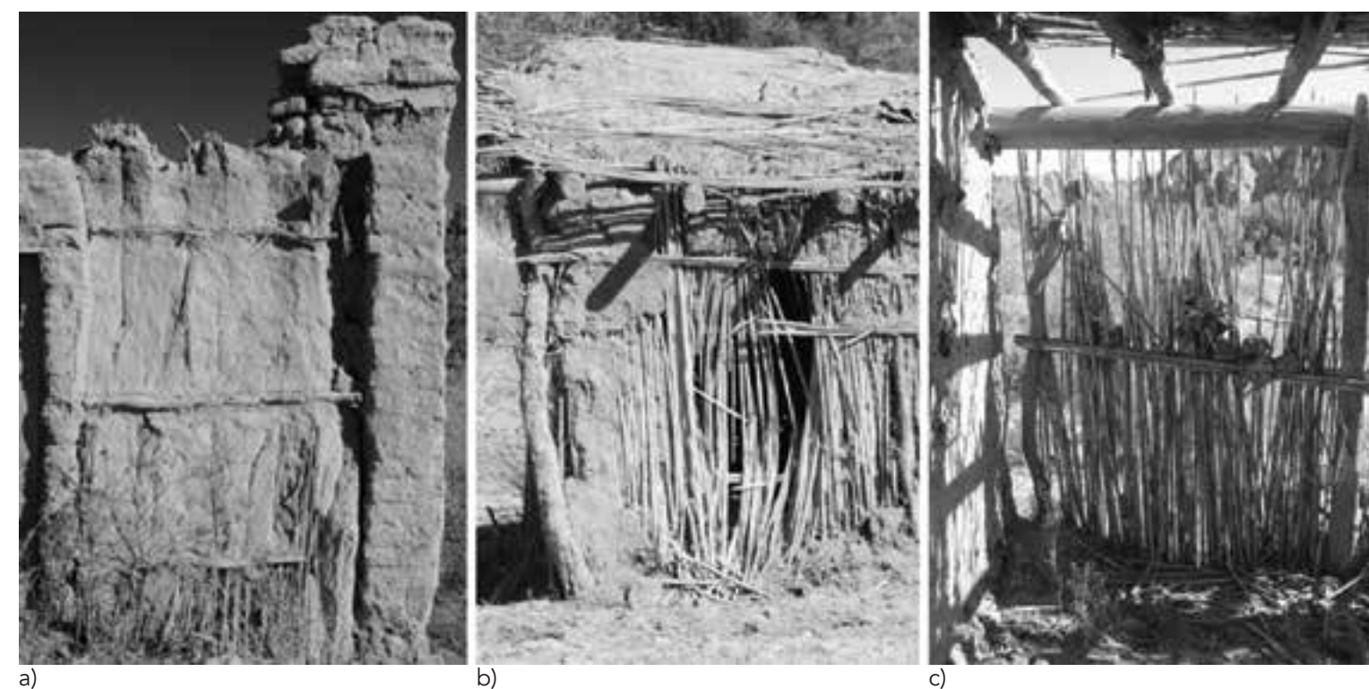
Fig.2 Quincha walls with Castile cane and carob lattice (credits: Guillermo Rolón, 2011)
