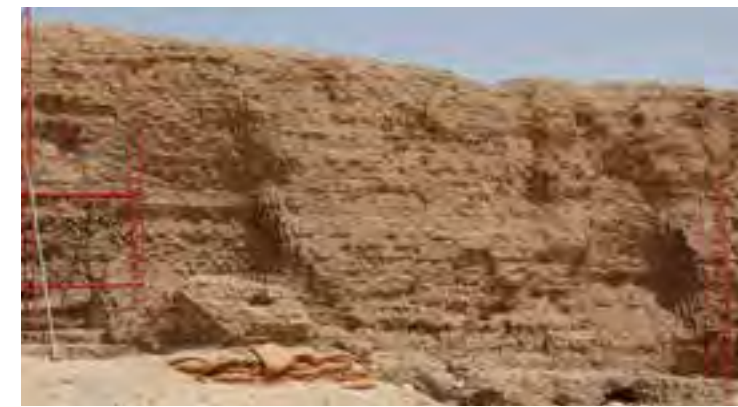
Fig.3 The west enclosure wall showing the completion of the stabilization of two collapsed areas where Coptic cells existed (credits: Anthony Crosby, 2006)
