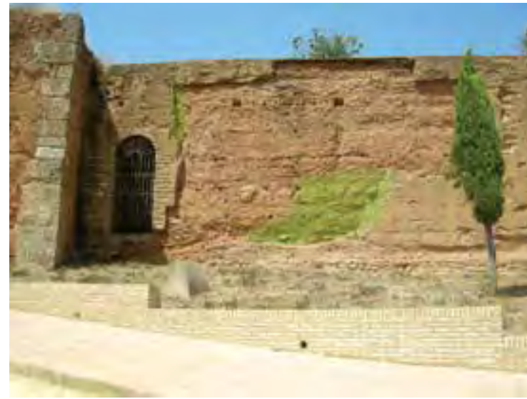
Fig.3 Damage in earthen the fabric of the wall between Towers 6 and 7 in 2009 (credits: A. González, 2009) Fig.4 Damage in earthen the fabric of the wall between Towers 6 and 7 in 2011 (credits: J. Canivell, 2011)
