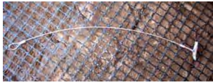
Fig.5 Aluminum wedges attached to stainless-steel cables used to attach geogrid to mud brick walls (credits: Anthony Crosby, 2010)
