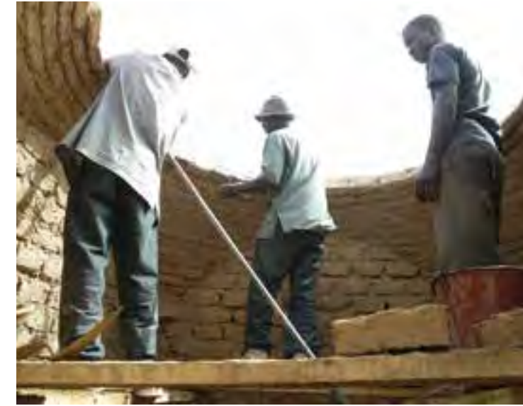
Fig.4 Construction of cupolas (credits: CRAterre, Laure Cornet, 2010)
