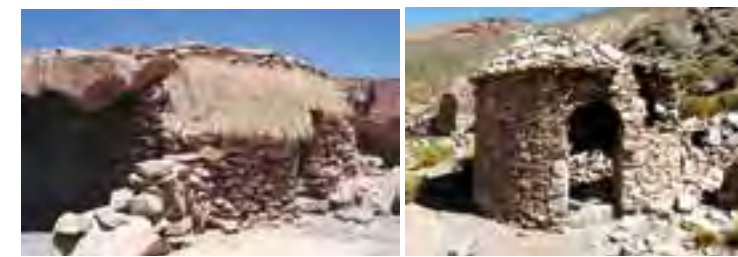
Fig.2 One puesto built with pirca seca (credits: Jorge Tomasí)
