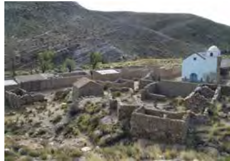
Fig.4 Hamlet and small church in La Cueva, Argentina, constructed of adobe, stone and clay, earthen plasters, and terracotta tiles roof (credits: Rodolfo Rotondaro, 2009)
