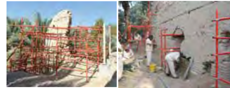
Fig.2 Al-Suroor Southern House after emergency stabilization (credits: Salman Muhammad © ADACH, 2011)
