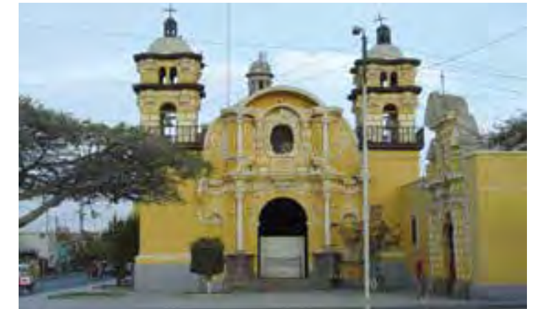
Fig.2 The Compañía Church, in Pisco: a) In 1920, the church had endured the great earthquakes of 1746 and 1877 without collapsing; b) By 2007, before the earthquake, the building had a cement floor, and the paved streets prevented earthen substrate from expelling vapor (credits: Domingo Canepa, 1920; Pedro Hurtado Valdez, 2007)
