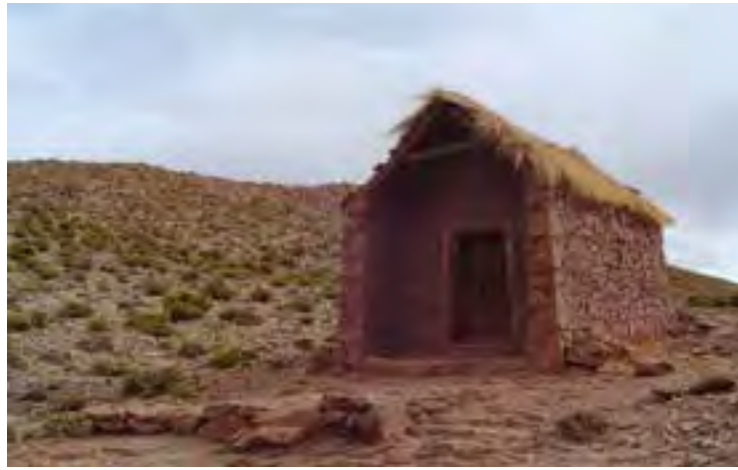
Fig.4 Domestic church (oratorio) with the guayado technique (credits: Jorge Tomasi)
