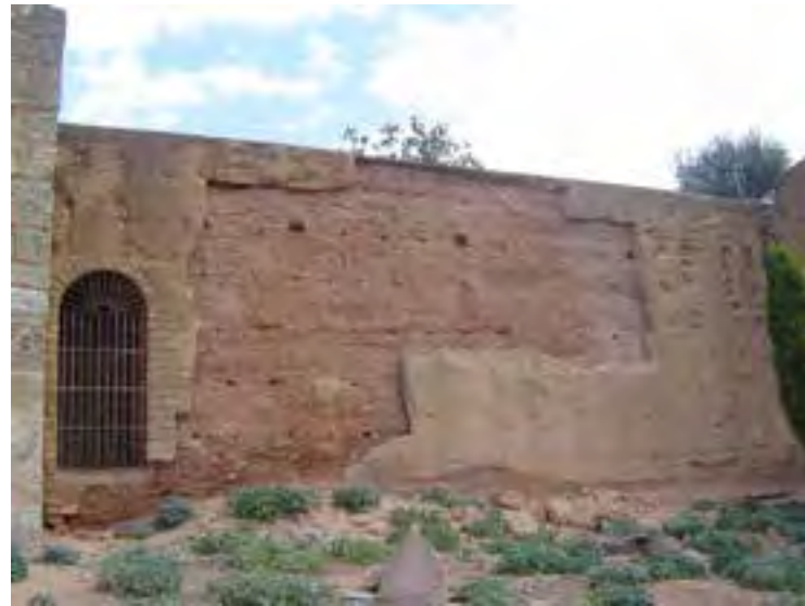
Fig.3 Damage in earthen the fabric of the wall between Towers 6 and 7 in 2009 (credits: A. González, 2009) Fig.4 Damage in earthen the fabric of the wall between Towers 6 and 7 in 2011 (credits: J. Canivell, 2011)
