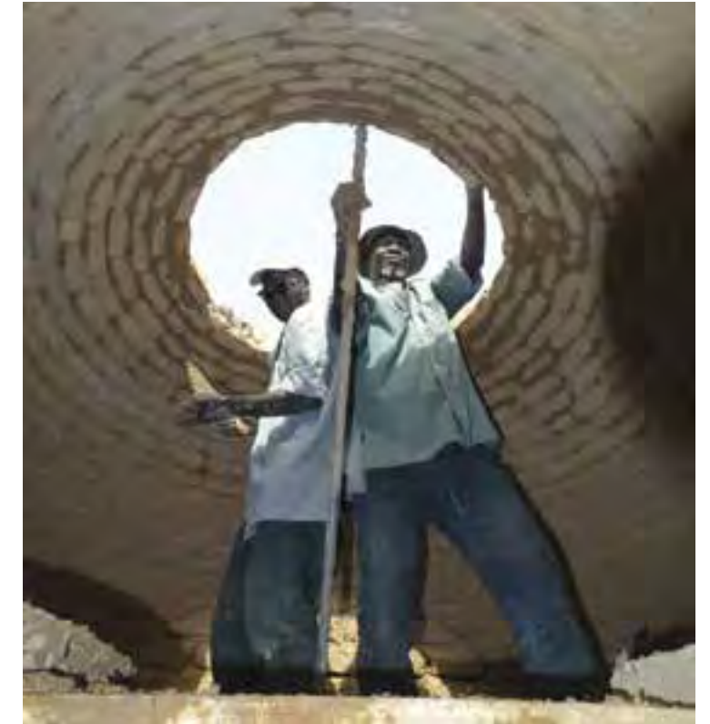
Fig.5 Construction of cupolas (credits: CRAterre, Laure Cornet, 2010)
