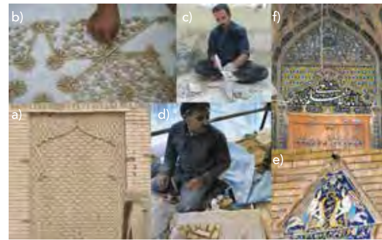
Fig.4 Examples of Moarraque, a method for surface protection of earthen architecture in Isfahan: a) brickwork in David's House; b), c) and d) design, cut and installation of mosaic pieces on earthen walls; diversity of approaches in the early 20th century in e) Sadr Madrasa and f) Harunieh alley (credits: Vahidzadeh et al., 2011)
