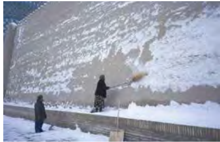
Fig.4 Traditional preventive measure of snow removal from a wall and wall base in Khiva, Uzbekistan (credits: Thierry Joffroy, 2003)
