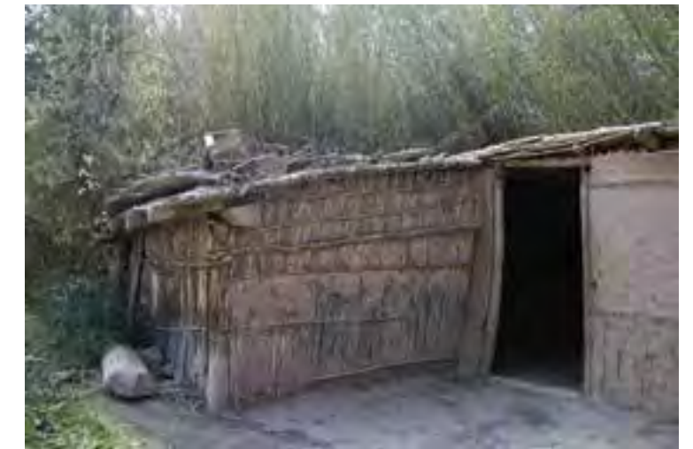
Fig.2 Quincha depot in an agricultural sugar plantation near Route 9, close to Maimará, Argentina (credits: Rodolfo Rotondaro, 2009)
