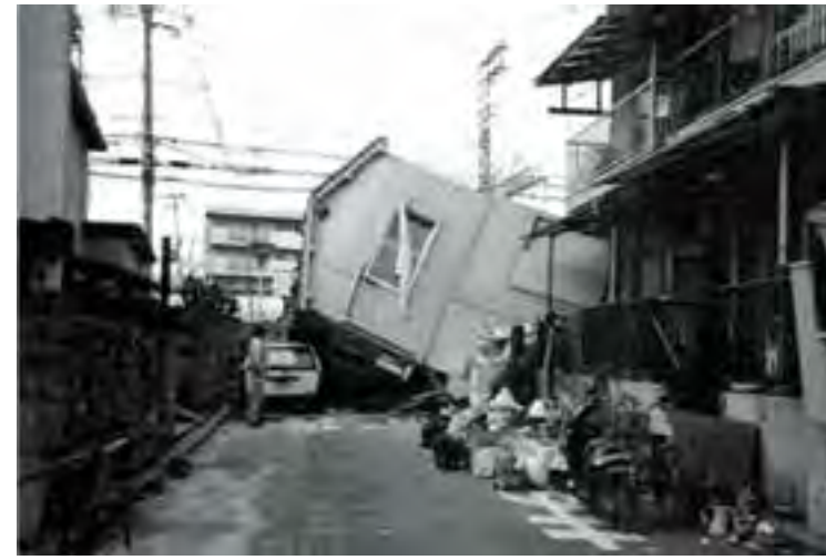
Fig.3 Kobe 15th Mansion (protected heritage) destroyed by Kobe Earthquake, M.7.3, January 17, 1995 caused liquefaction of the ground (credits: K.Masuda 1995)
