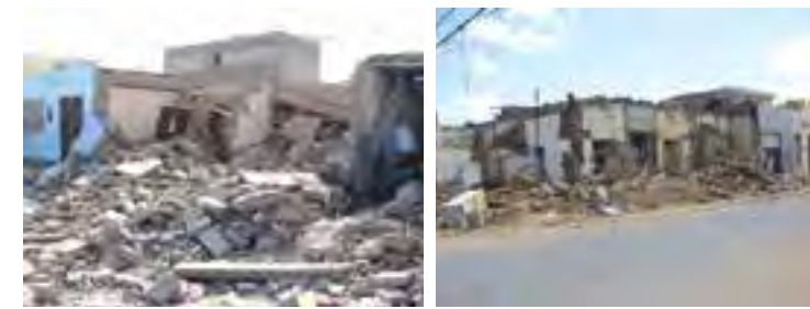
Fig.1 Collapsed houses during the earthquakes of Pisco, Peru, 2007 and Maule, Chile, 2010 (credits: J. Vargas-Neumann, 2007 y 2010)
