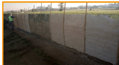
Figure 5 – Render panels over adobe wall
