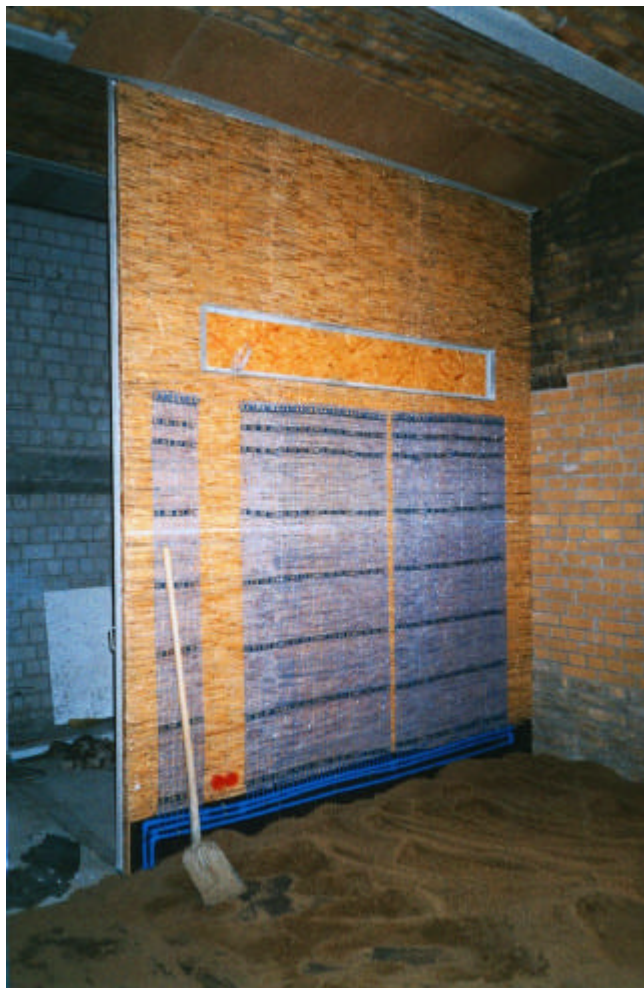
Picture 1: Preparation of a wall-heating-system
