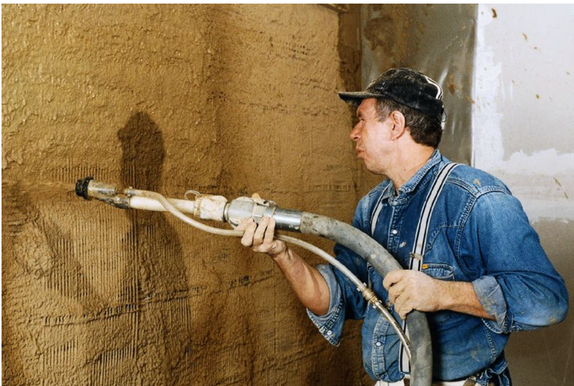
Picture 4: A vocational training in earthen plasters
