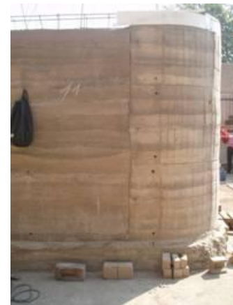
(Fig. 3) Junta constructiva vertical
