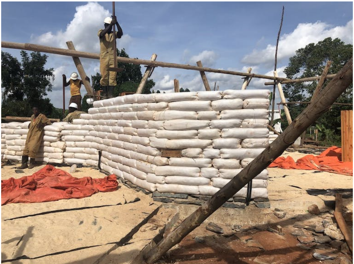
Figura 24 – Terra ensacada na Escola Mustardseed, Uganda (Acervo Will Boase Photography)
